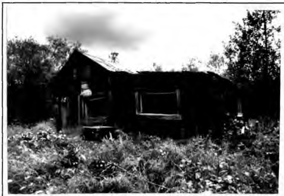
Figure 77. The Remington/Duffy/Baquir House, 1993. The view is looking southwest.
